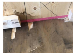
Fig. 8. Sample taken from the top side of the floor structure (CLT) under the sound and vibration pads and inner walls (CLT). The surfaces have been stained primarily by discoloured water.
