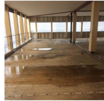
Fig. 5. On several occasions, water pooled on the floor structure. Precipitation ran down primarily from the above floor structures.
